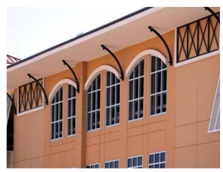
The precast concrete panels were cast with embedded thin brick, cast-in tile mosaics and rustications, with a number of paint colors used. Some were used to create false windows cast into the panels (lower row). These variations were embellished with accessories such as decorative grilles and awnings.
